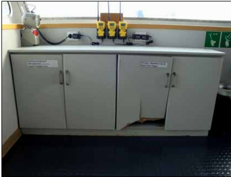
Figure 6: Impact damage to cabinet 16
