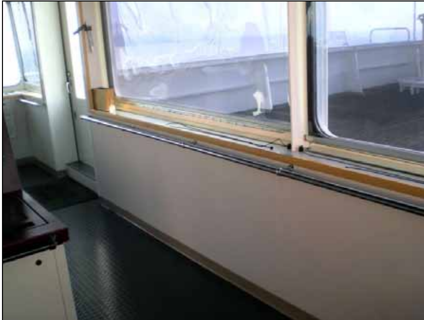
Figure 47: Handrail on the port side of the bridge
