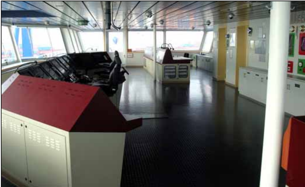
Figure 20: No handrails at the aft end and starboard side of the bridge
