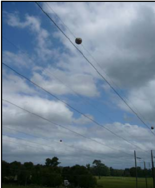
Figure 15: Example of wire markers mounted on a multi-strand powerline
