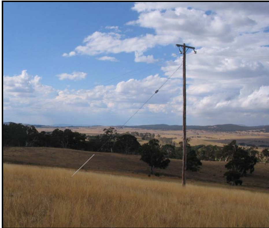
Figure 11: Example of a guy wire
