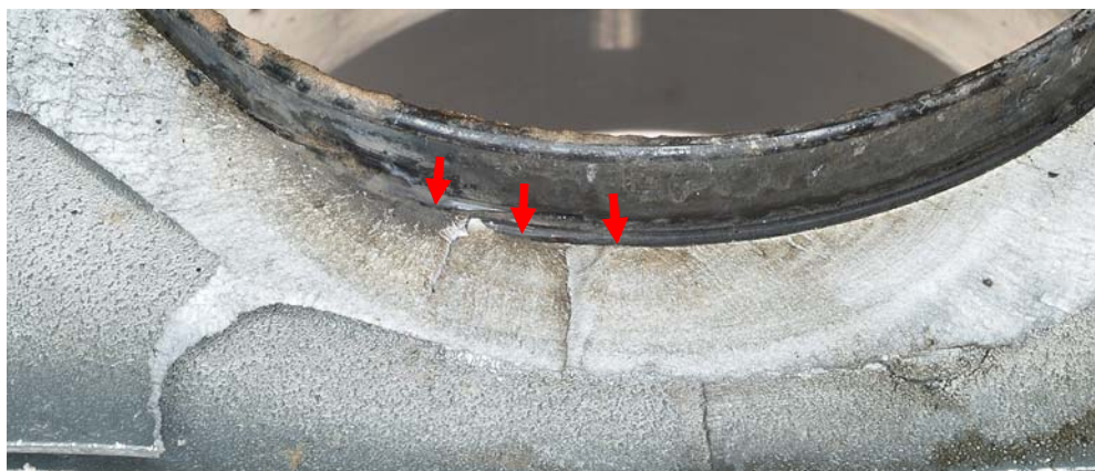
Figure 8.66: Fatigue cracking features, occurrence 2001/2885, VH-MJA
