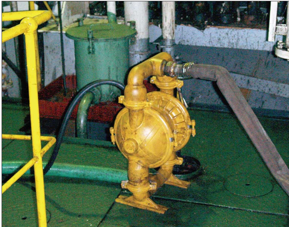
FIGURE 4: Air-operated pump
