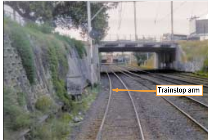
FIGURE 8. The cutting approaching signal W 223
