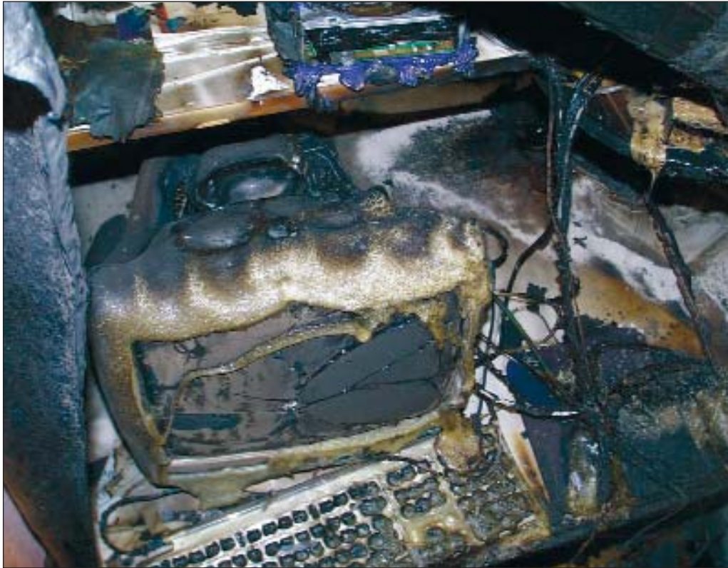
FIGURE 7: Fire damage to computer workstation
