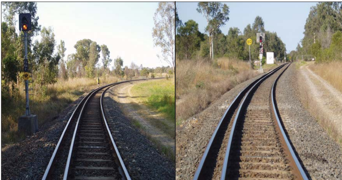
FIGURE 4: Signal FS66P (left photograph), 360 metre radius curve, signal FS66 (right photograph)
