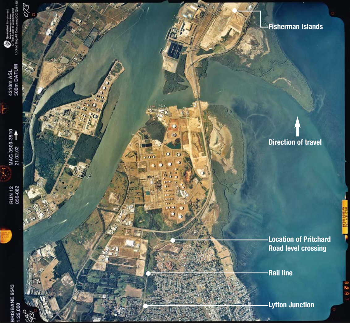
FIGURE 1: Aerial photograph of Fisherman Islands precinct
