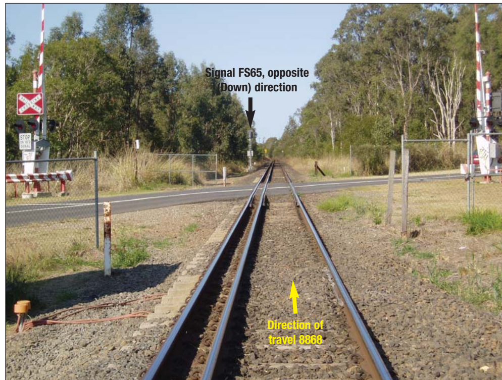
FIGURE 8: Pritchard Road level crossing
