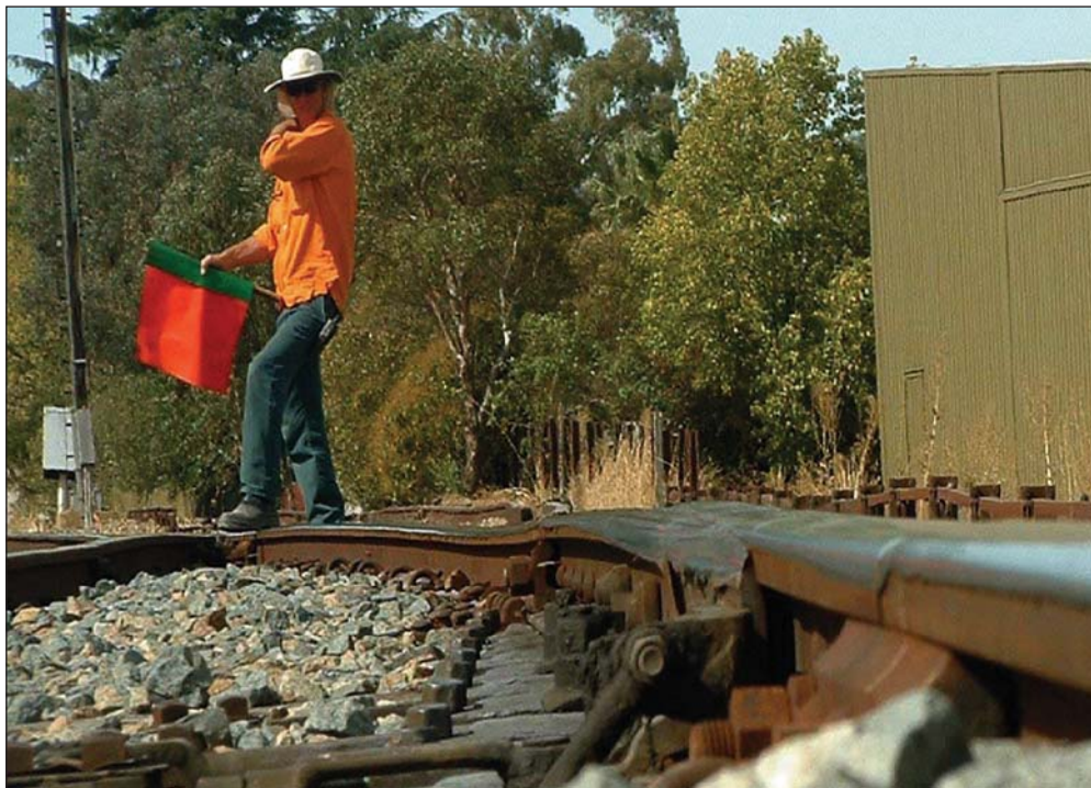
FIGURE 29: Vertical profile, illustrating the undulations of the curved closure rail and the flared rail at the point blade
