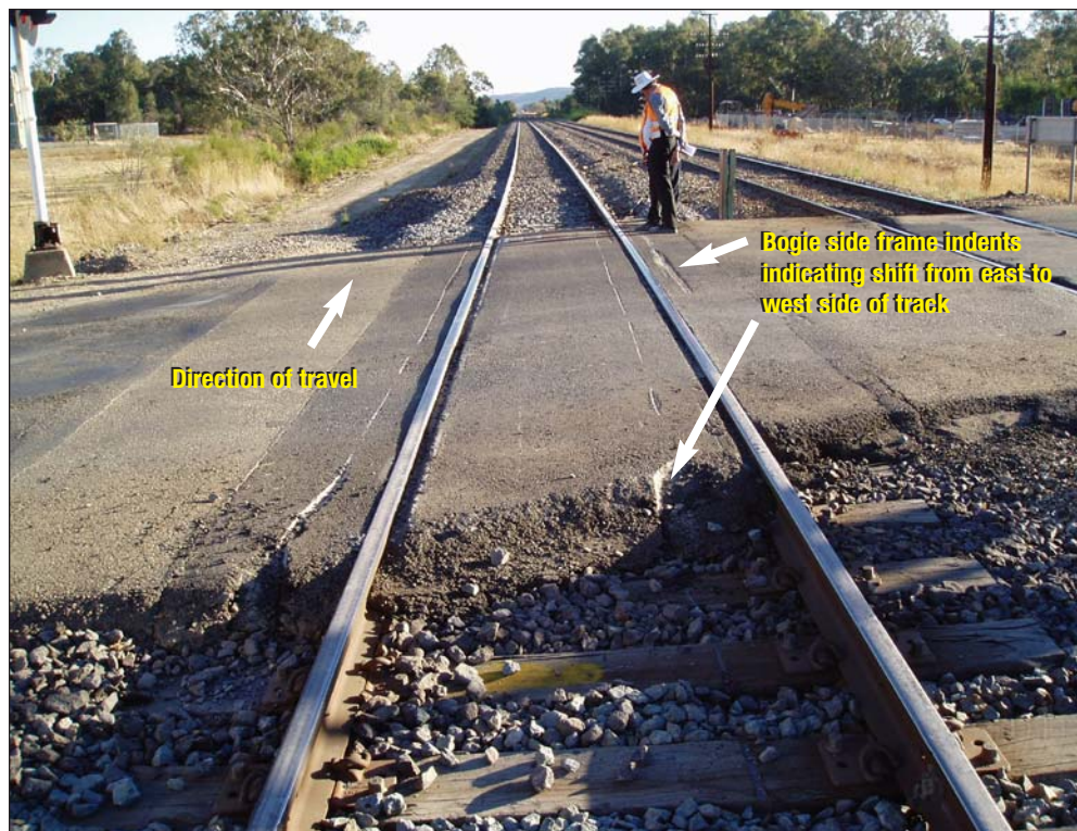
FIGURE 4: Shanley Street level crossing, looking south
