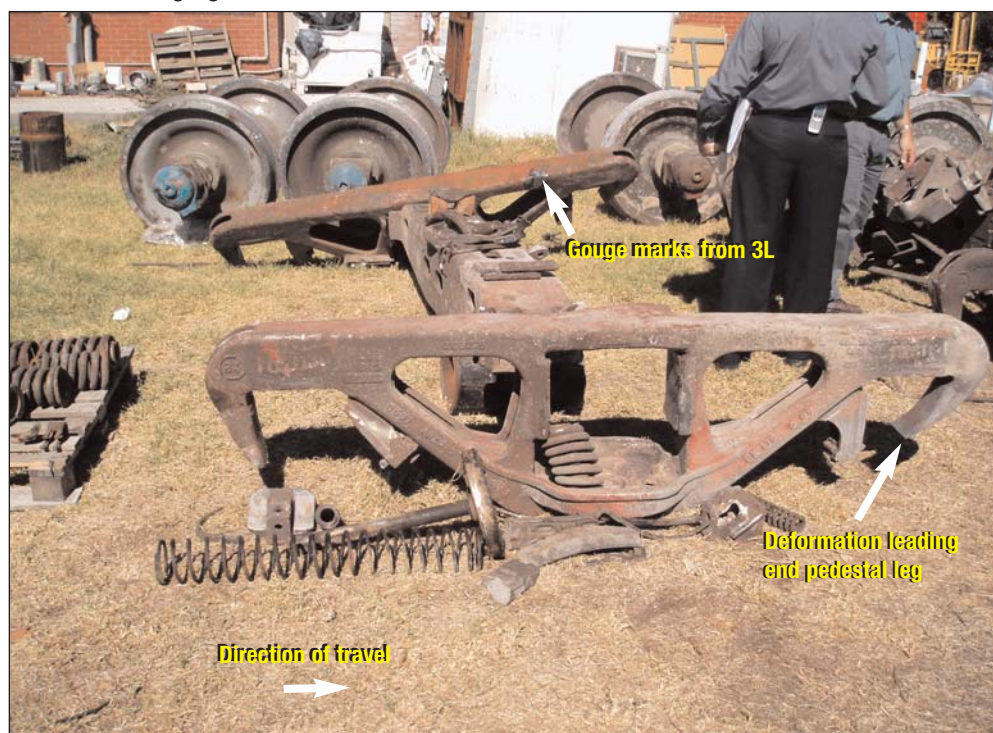
FIGURE 11: Recovered components of bogie VXSC 15611 showing deformation of leading pedestal leg and gouge marks from wheel 3L
