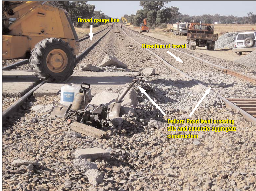
FIGURE 7: Dellaro Road level crossing under repair
