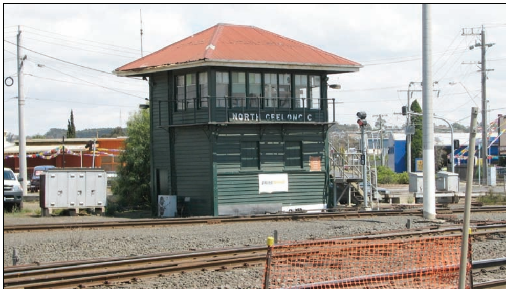
Figure 1: View of the North Geelong 'C' Signalbox
