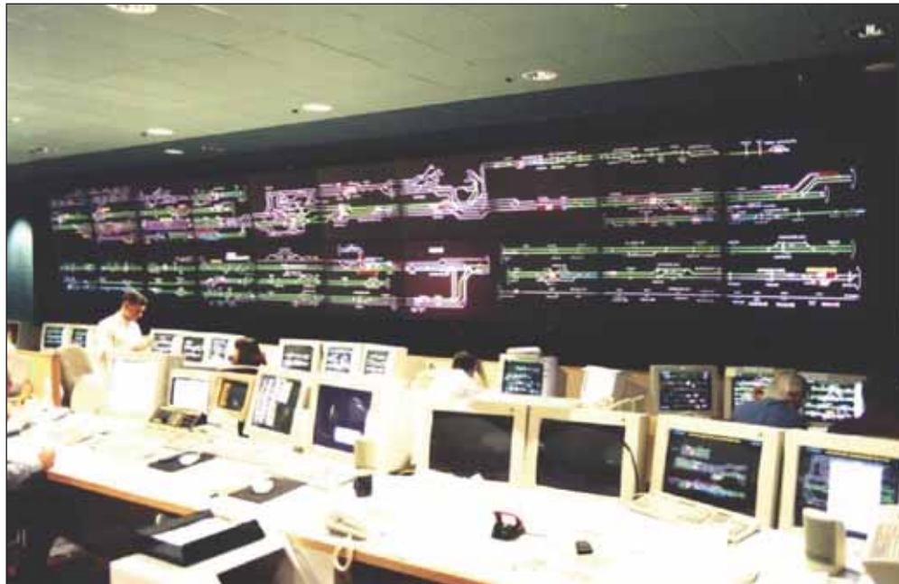
FIGURE 4: Mayne Control Centre showing overview screen and individual UTC workstations in the foreground
