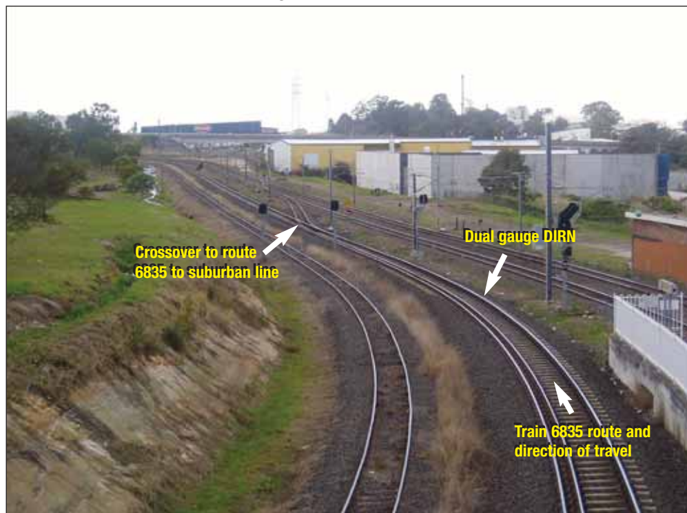
FIGURE 1: Crossover at Murarrie looking east
