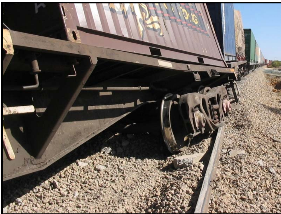
Figure 20: Damaged sleepers and spread gauge
