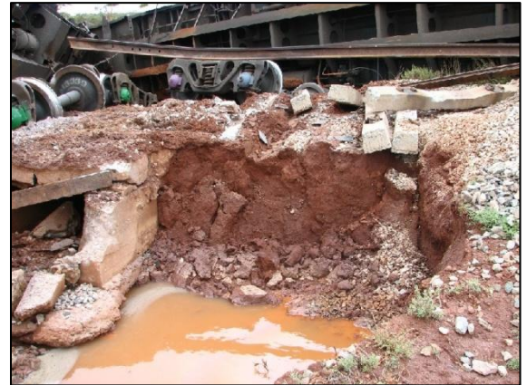
Figure 8: Culvert at derailment site
