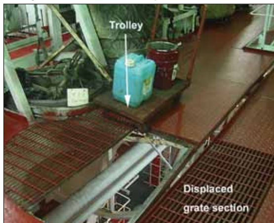
FIGURE 2: Deck grate and hole immediately after the accident
