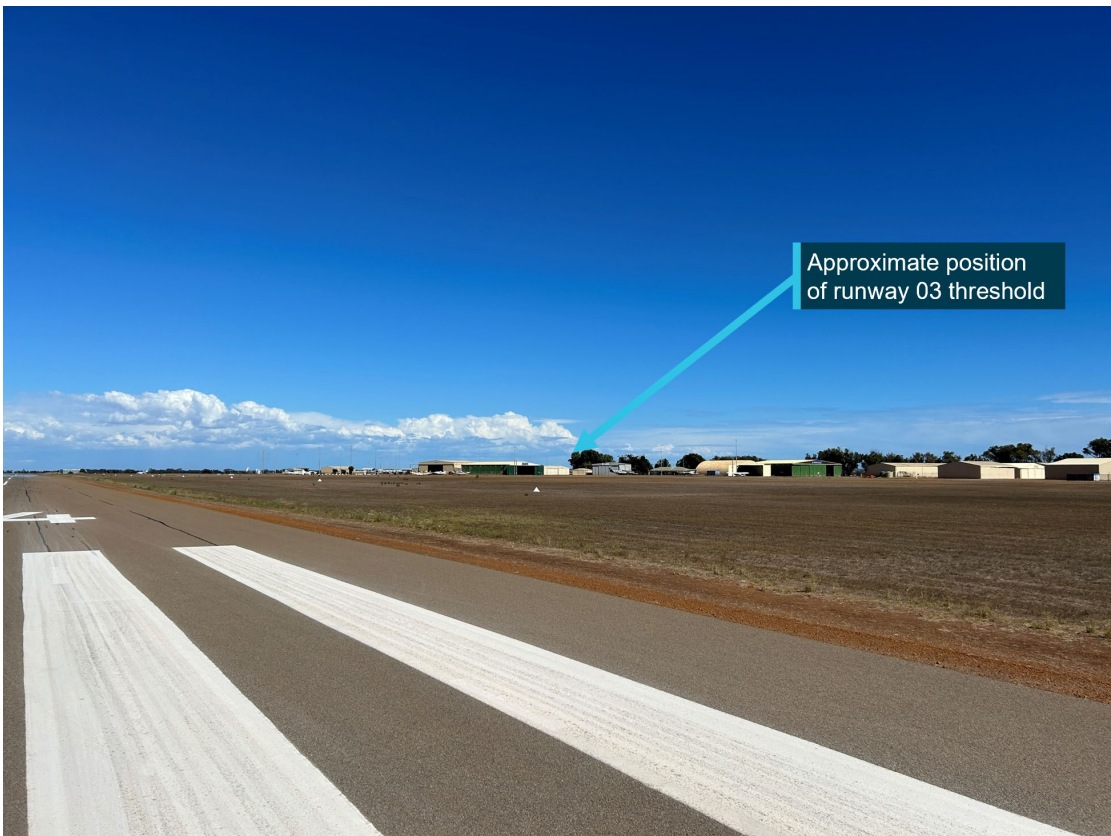
Figure 4: View of runway 03 threshold from runway 14 threshold
