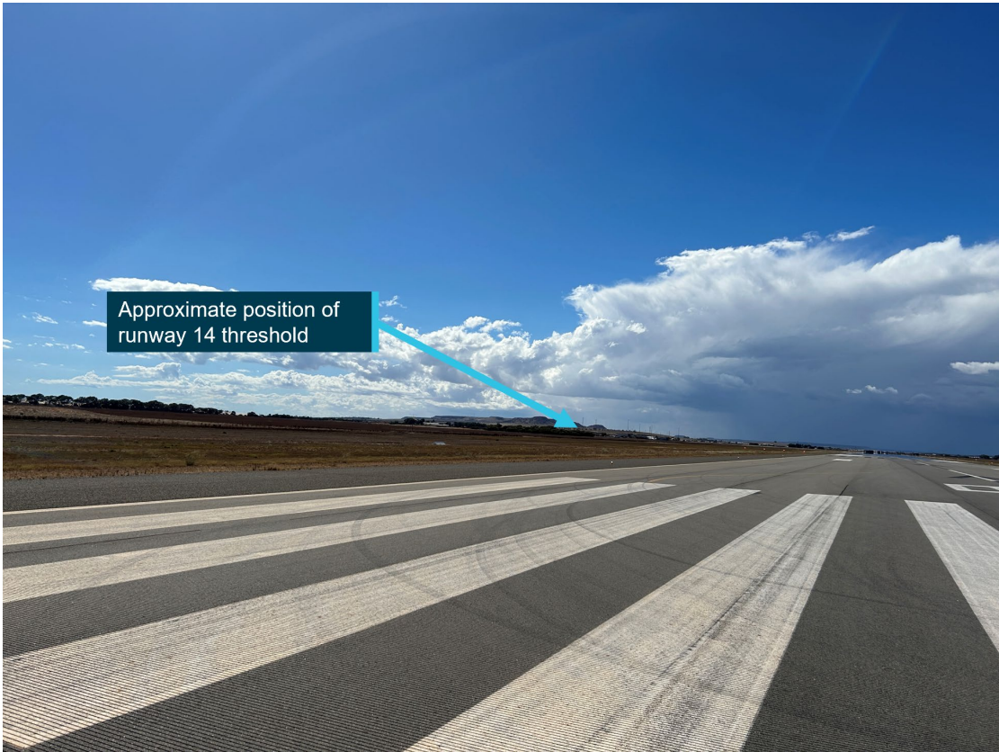
Figure 3: View of runway 14 threshold from runway 03 threshold
