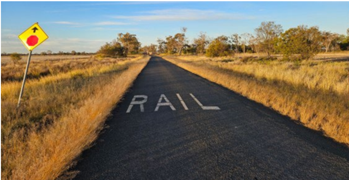
Figure 7: First advance warning, northern approach
