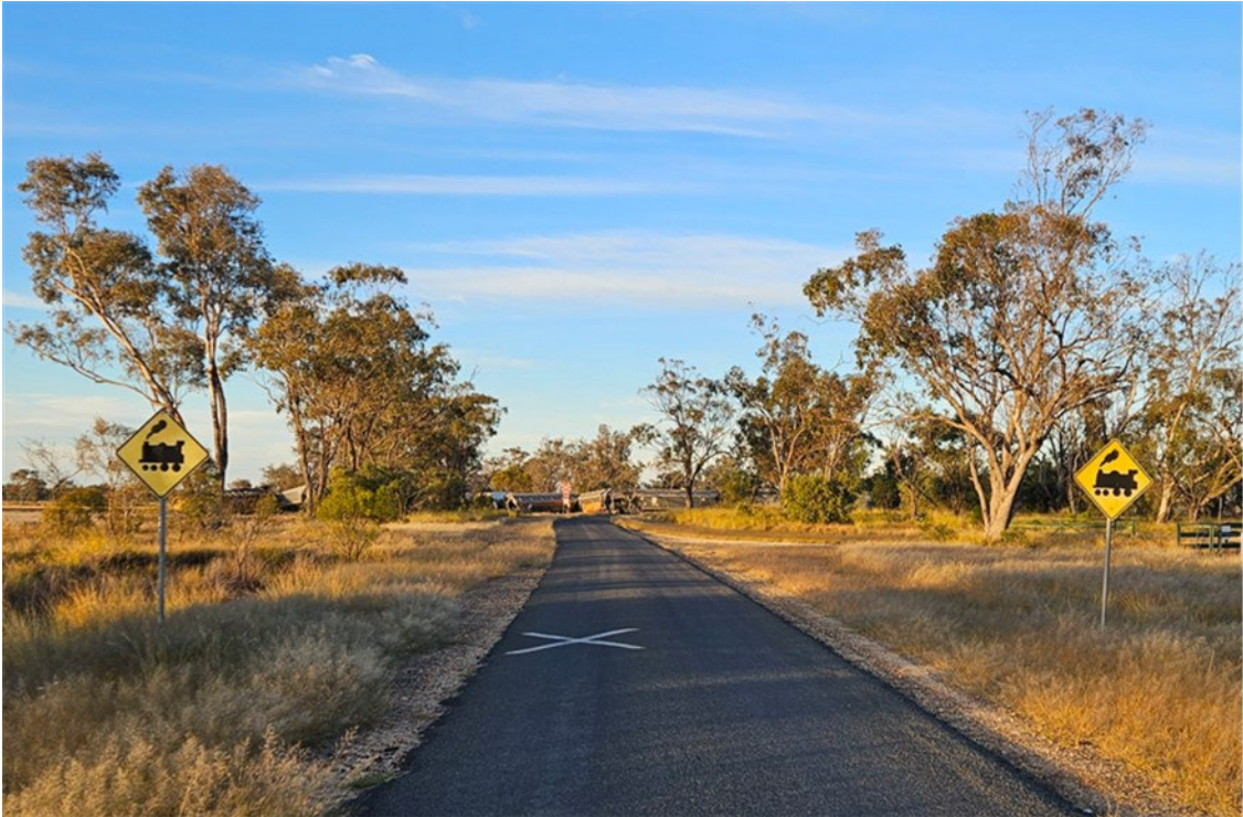
Figure 8: Second advance warning, northern approach
