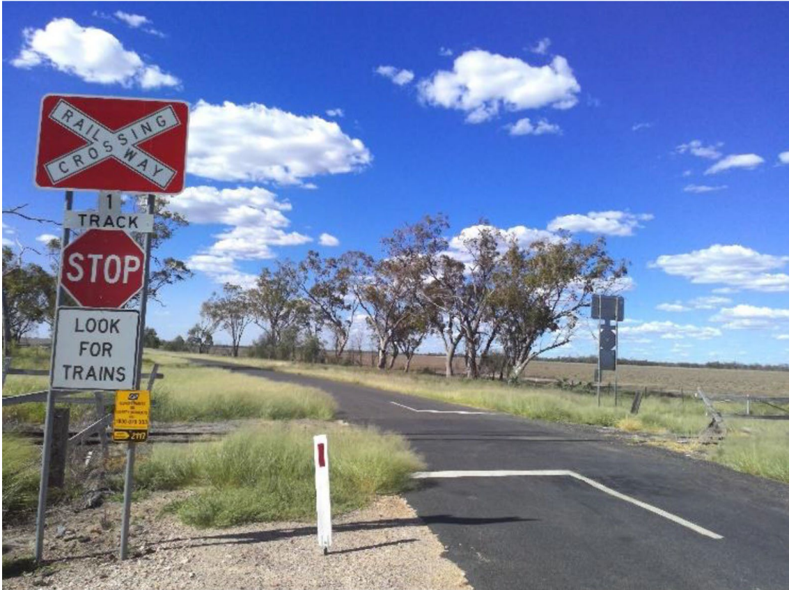
Figure 9: Stop sign assembly and stop line, northern approach
