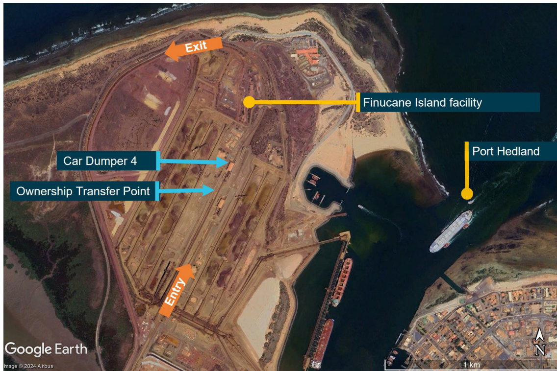
Figure 1: Finucane Island facility showing car dumper 4 and its owner transfer point
