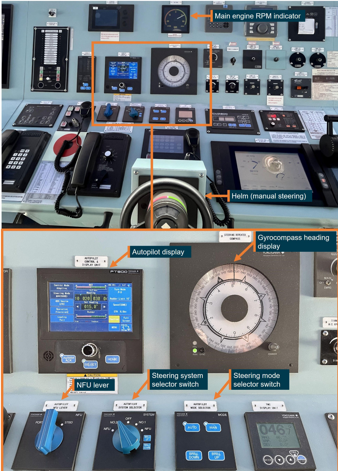
Figure 6: Hagen Oldendorff's bridge console layout showing steering mode controls
