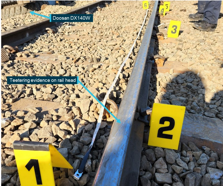
Figure 5: Teetering evidence on the rail head
