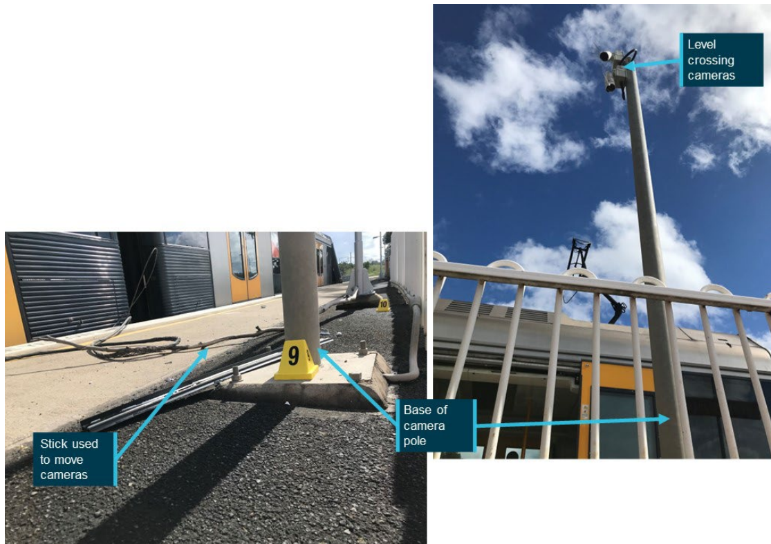
CCTV cameras facing the ground and away from the level crossing, moved by the convicted felon as captured on CCTV. Source: OTSI
