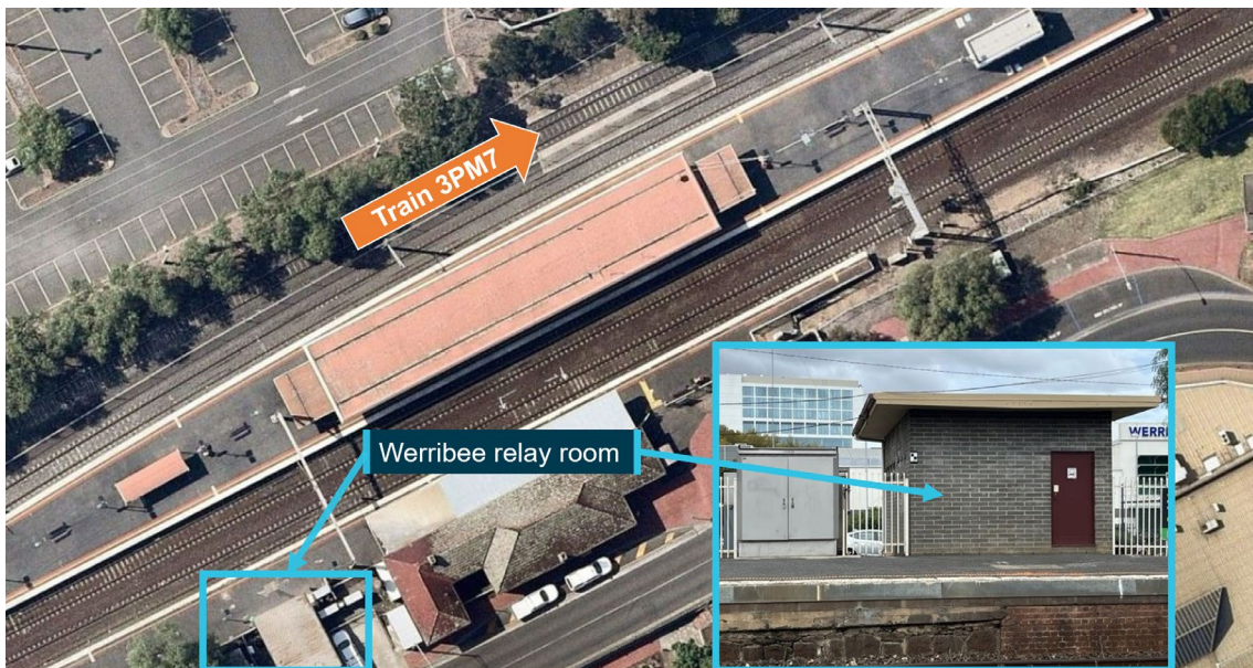
Figure 10: Aerial view of Werribee Railway Station and relay room
