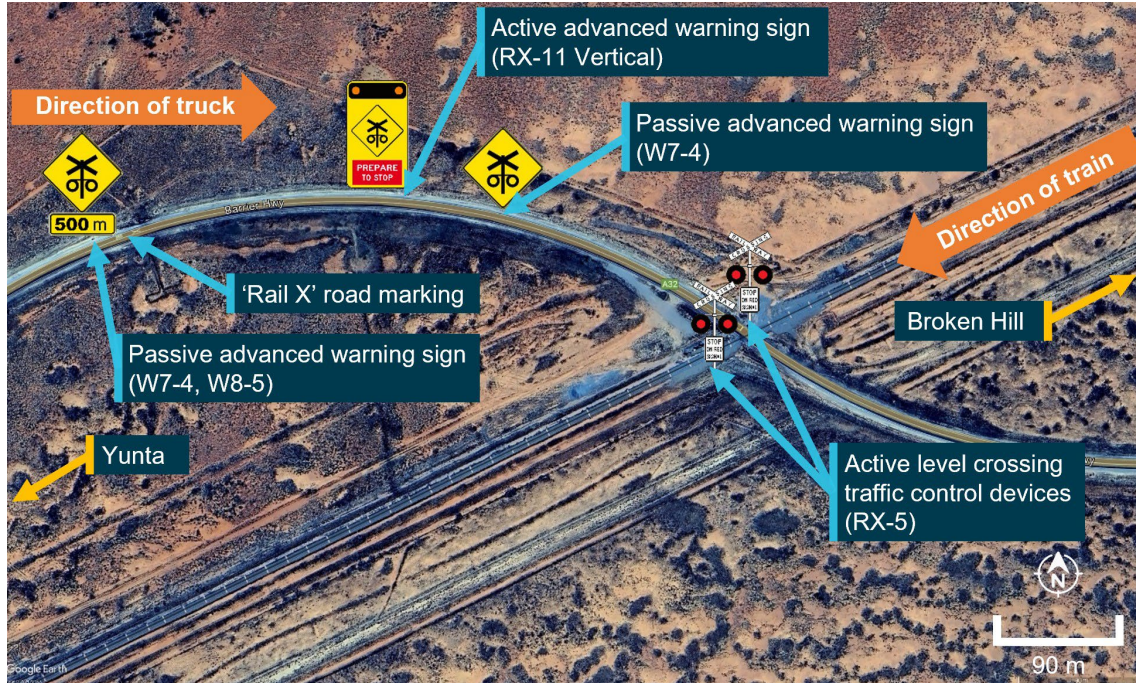
Figure 4: Aerial view of the level crossing approach and road alignment
