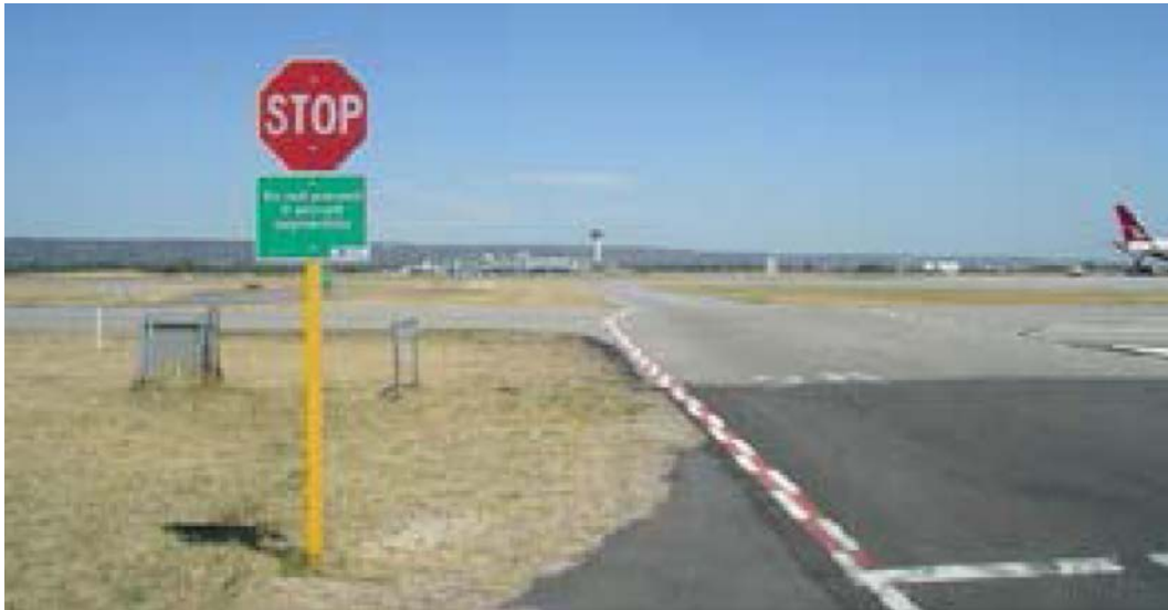
Figure 2: Photo showing stop sign and red and white zipper markings that denote a taxiway like that for taxiway R
