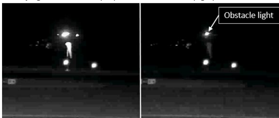
Figure 4: Flashing primary wind indicator showing the windsock illuminated when the runway lights were active (left) and not illuminated (right)
