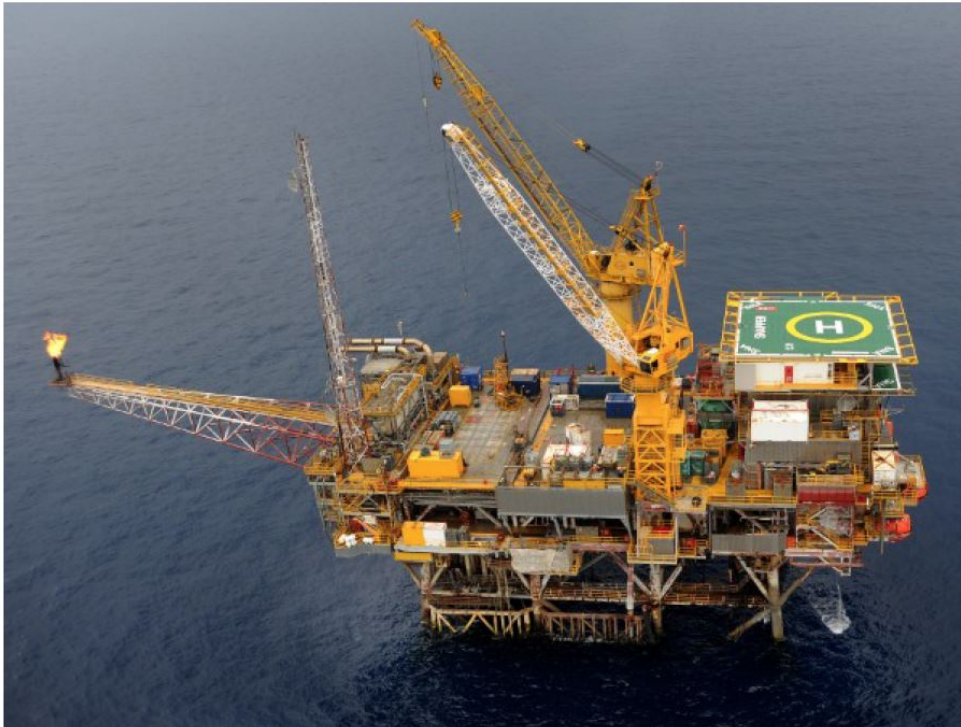
Figure 6: Snapper platform and helideck, looking east
