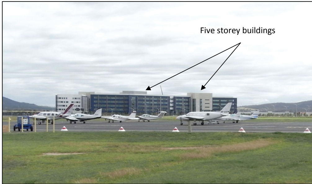
Figure 3: Ground-based view of the adjacent buildings from the southern side of runway 12
