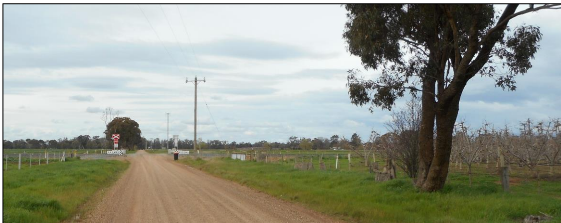
Figure 2: Pogue Road approach to the level crossing. The view to a train approaching from the right was obscured by road-side vegetation and an orchard.
