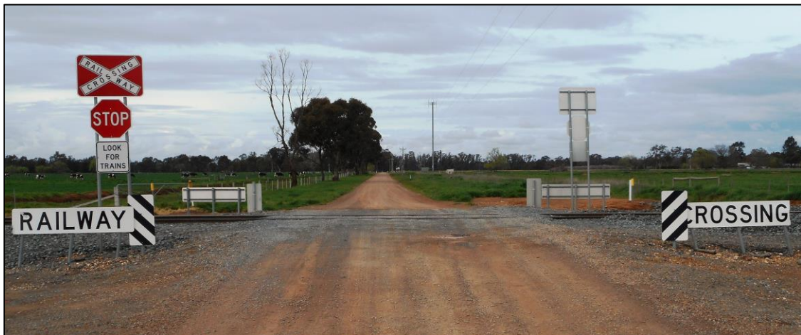
Figure 1: Pogue Road level crossing viewed from the direction of the car’s approach
