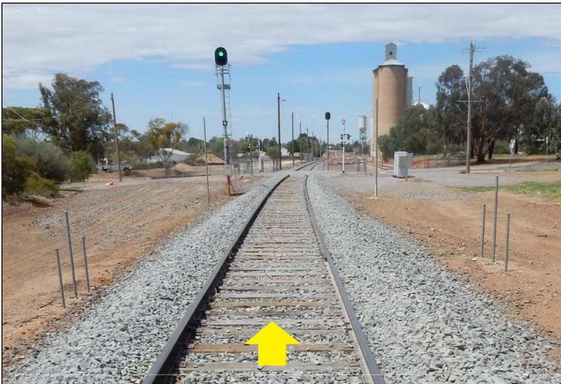
Figure 4: Approach to the William Street level crossing from Carwarp. The photograph was taken after track restoration that did not include the turnout on the Melbourne side of the crossing.
