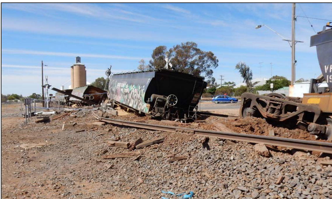
Figure 3: Track damage on the approach side of the William Street level crossing
