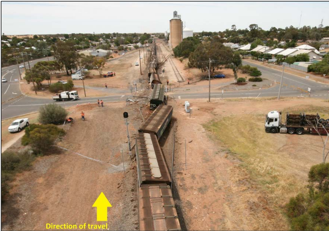
Figure 2: View of derailed train at the William Street level crossing.
