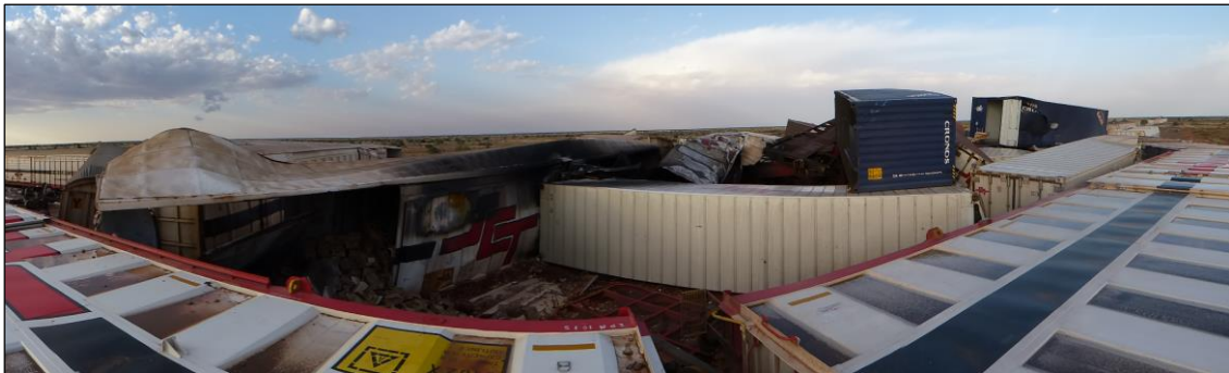
Figure 3: Panoramic view of derailed vehicles and containers
