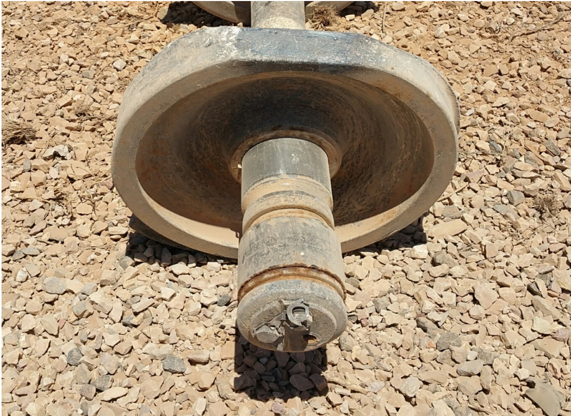
Figure 7 shows that the end seals of the bearing appearing to be ‘wet’ which indicates that some grease may have been liberated during the derailment. This also indicates that there may have been a failure in the bearing seal. Source: Genesee & Wyoming Australia
