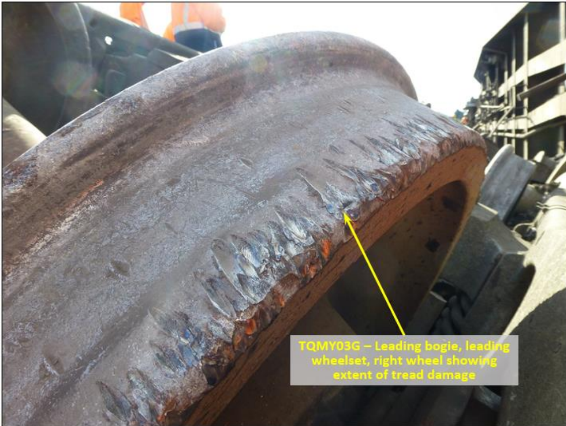
Figure 5: TQMY03G – Leading bogie, leading wheelset, right wheel (direction of train travel) showing evidence of extensive of tread damage
