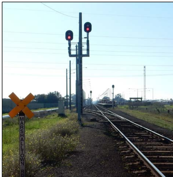
Figure 10: Multiple route two-position signal MSL26, with two light signals.
