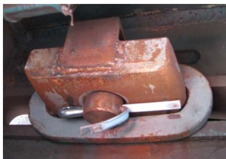
Figure 18: Welded angle retainer
