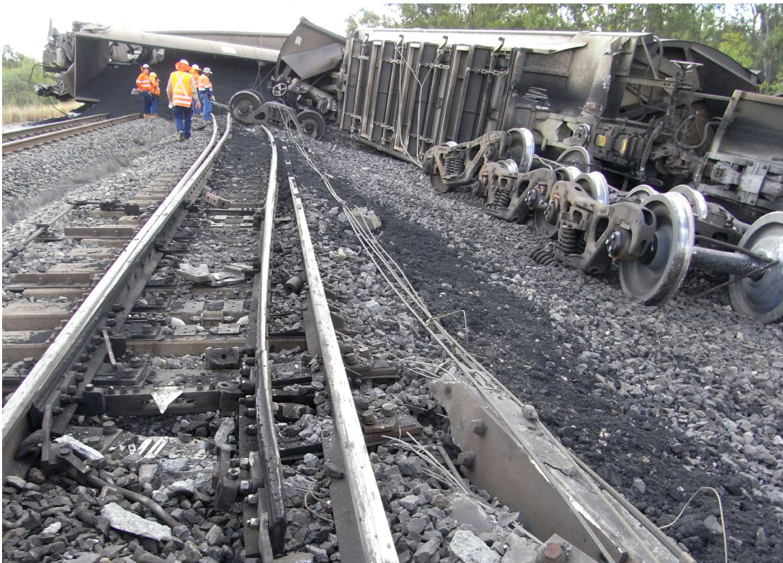
Figure 11: Duaringa derailment site
