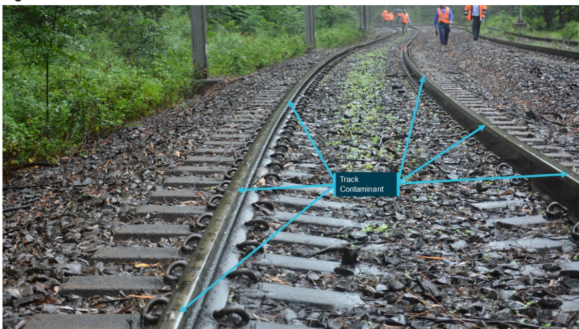
Figure 11: Close up of track contaminant at 94.000 km
