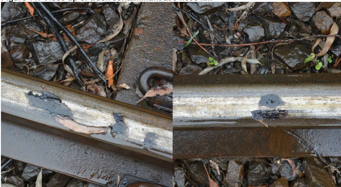
Figure 11: Close up of track contaminant at 94.000 km
