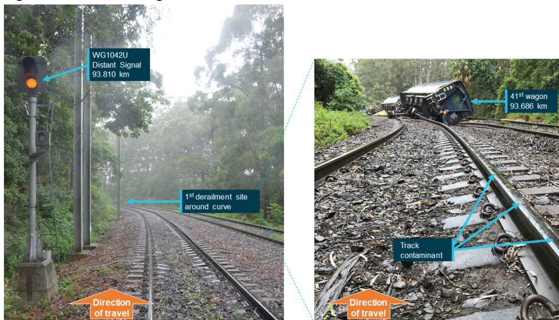
Figure 7: Rail line leading to first derailment site
