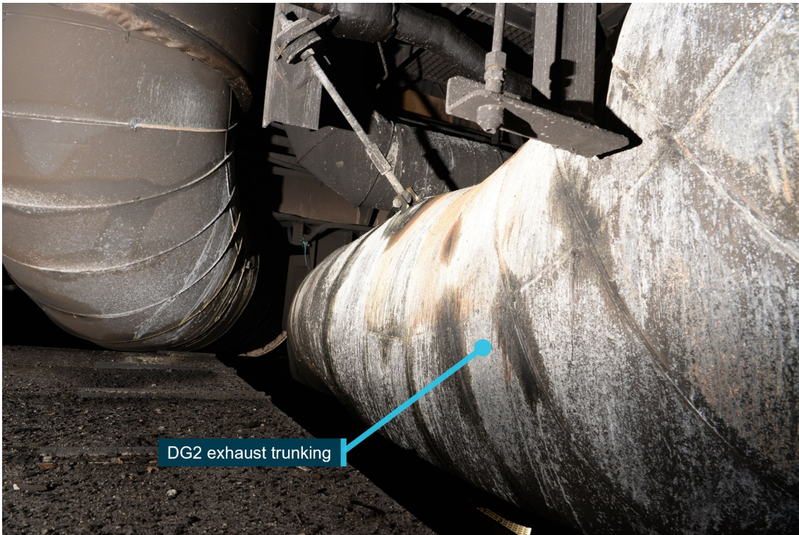
Figure 19: Upper surfaces of DG2 exhaust trunking
