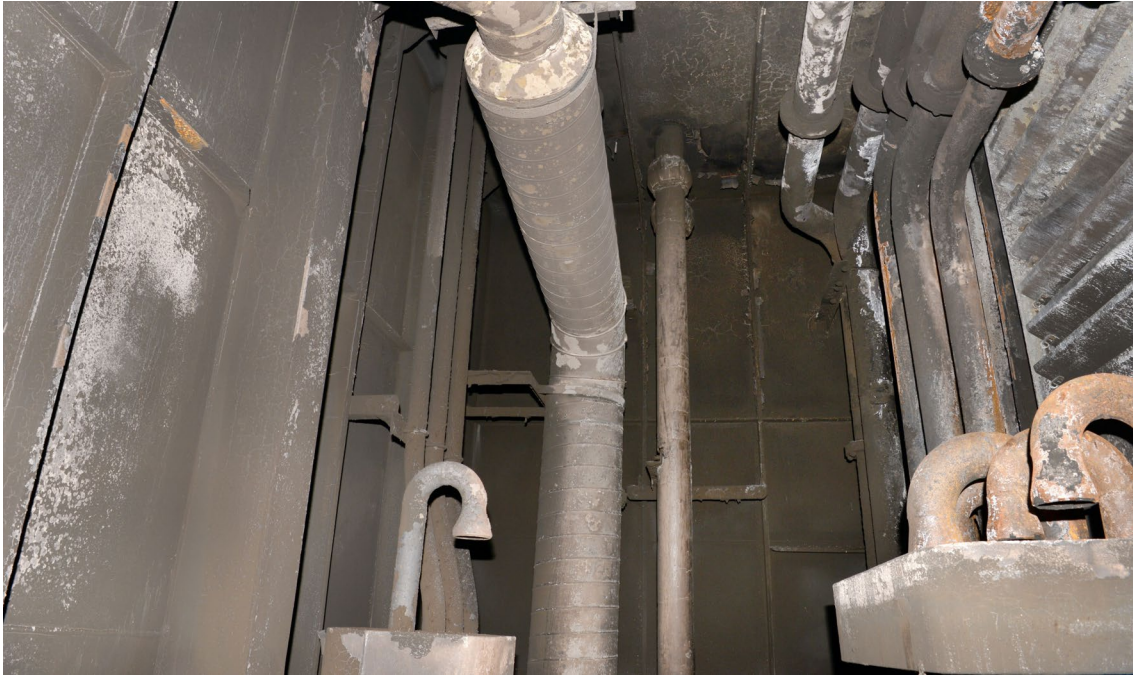
Figure 25: Interior of exhaust ventilation casing (upper level)
