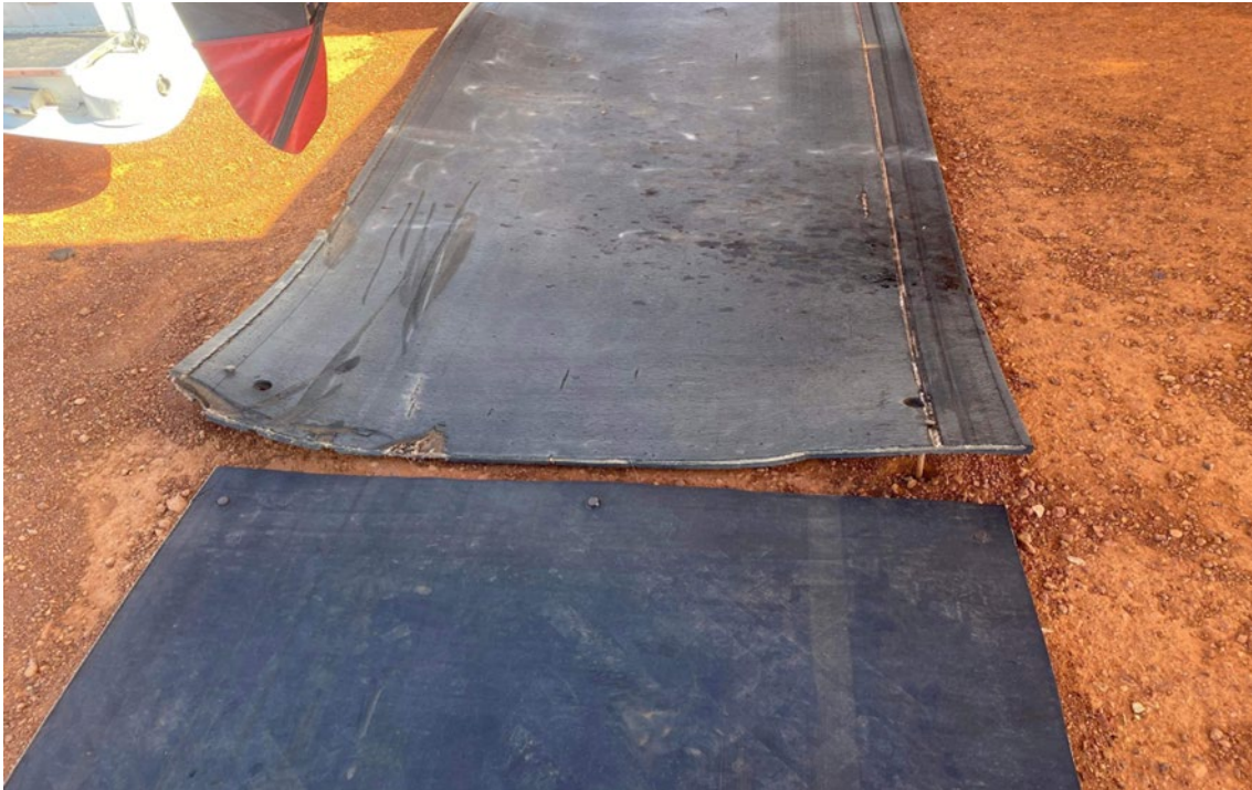
Figure 2: Dislodged inner matting
