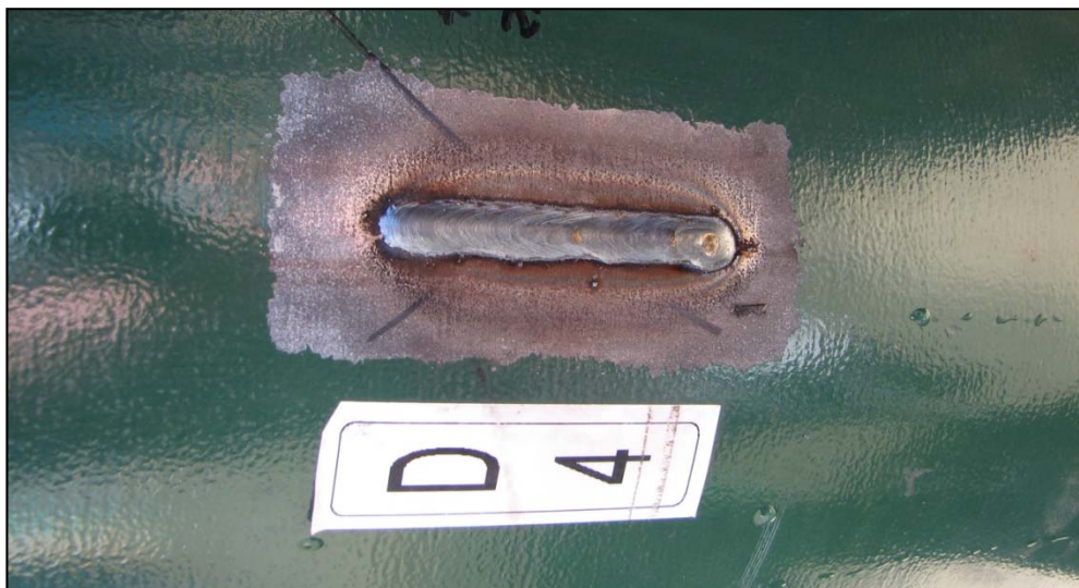
Figure A6: Flaw D4, after failure by leaking and over-welding in preparation for subsequent tests
