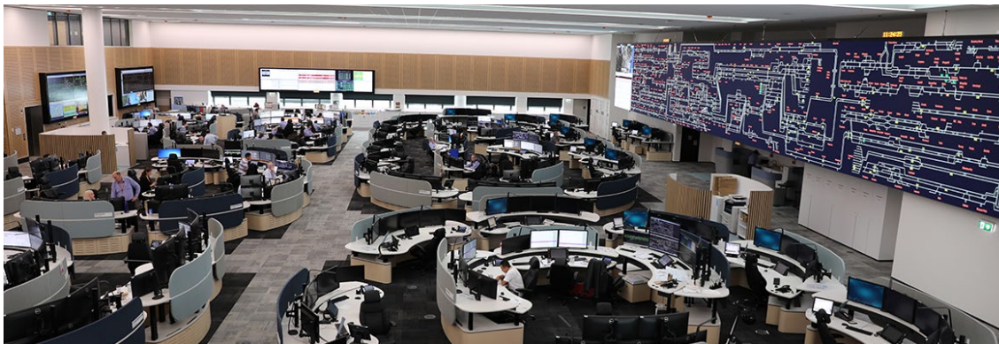
Figure 2 Rail Operations Centre (ROC) control room
