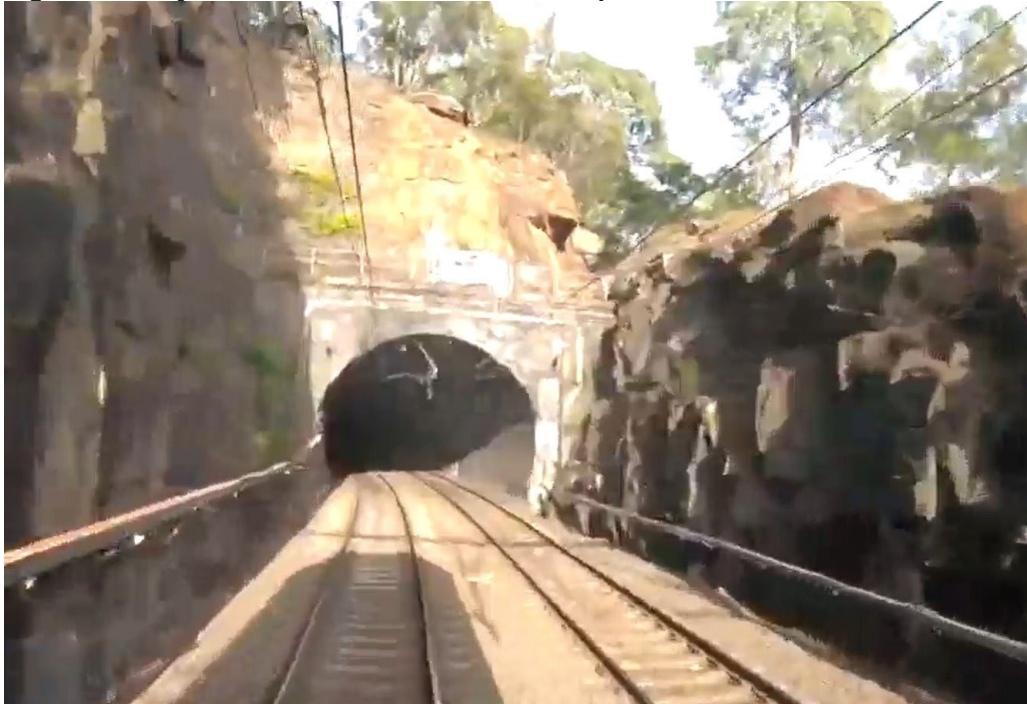
Figure 3: Entry to Boronia Tunnel No. 3 in the up direction
