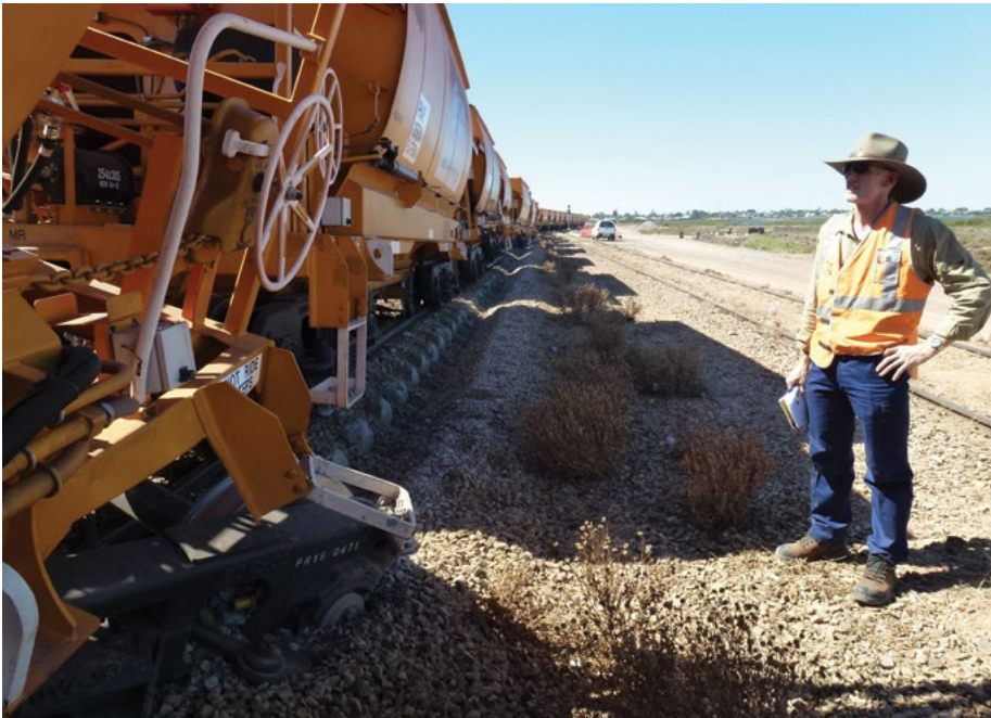
Figure 6: An ATSB rail investigator at work
